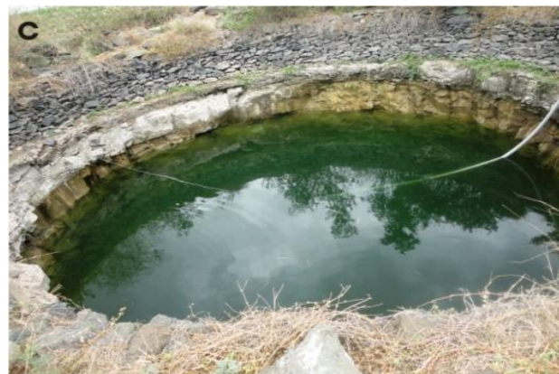
Fig 4: Field photographs of water abstraction structures (dug wells) from the study area.
