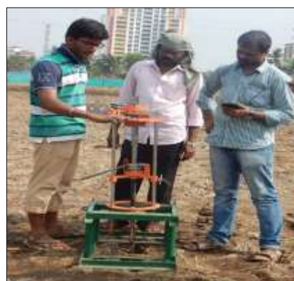
Fig 1: In-situ measurement of shear strength
