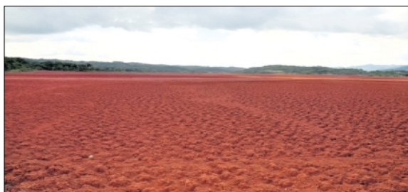
Fig 3: Disposal of red mud by dry stacking method.
